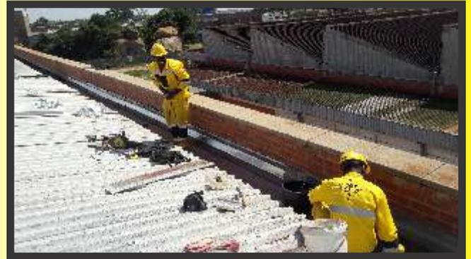
**LAPF pension fund (Toyota Zimbabwe):** The rainy season had become unbearable for our client due to leaks in their premise` roof and gutters. We replaced their old gutters and carried out all necessary roof repairs s that they would carry out their operations without having to worry about their equipment being damaged due to the rains
